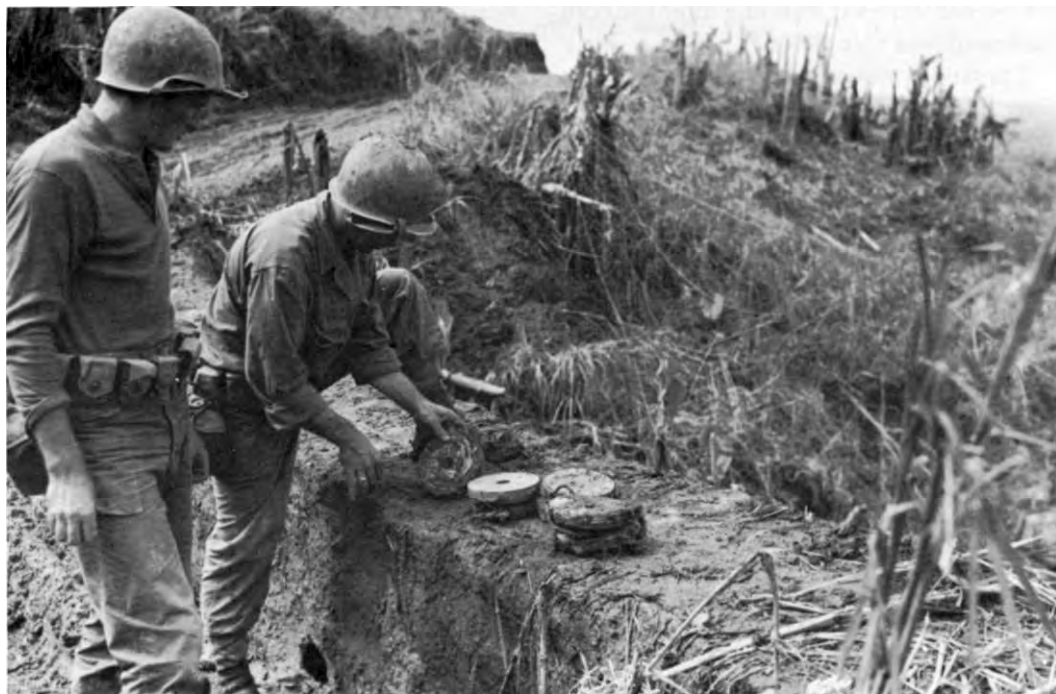
ENGINEERS REMOVE LAND MINES from a bridge on Breakneck Ridge.
