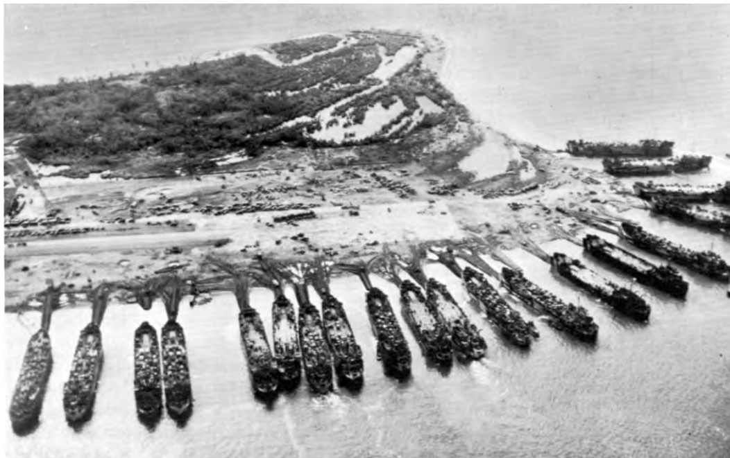
LST'S UNLOADING AT TACLOBAN AIRFIELD. The causeways leading from the beach to the ships were built by bulldozers scraping sand and earth to each ship as it landed.
