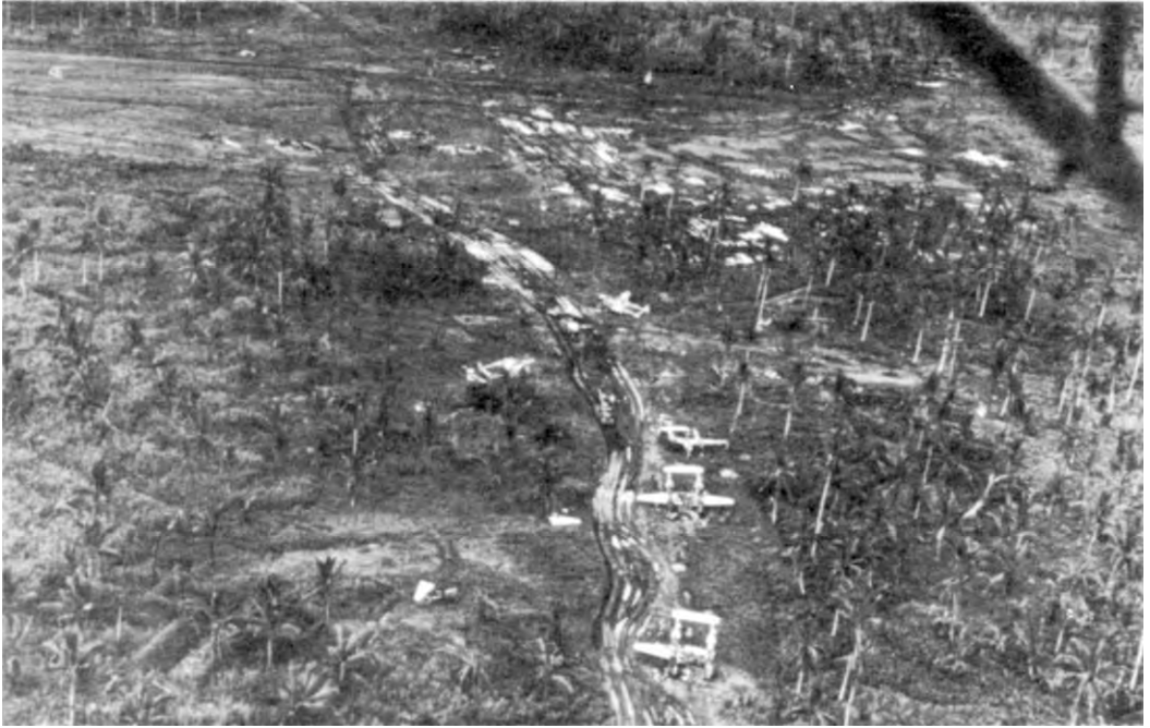
OPERATIONAL LOSSES AT THE BURAUEN AIRFIELDS forced their abandonment and the construction of the field at Tanauan.
